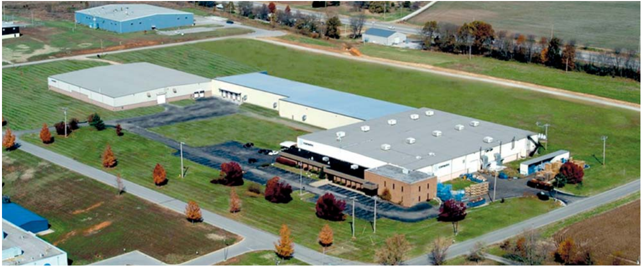
COMEFRI USA: Manufacturing and Warehouse facilities in Hopkinsville, KY. Total facility: 125,000 sq.ft. Producing centrifugal fans for the HVAC industry.
